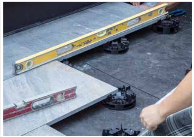
The BlackJack® Pedestal System ensures a perfectly level surface.
