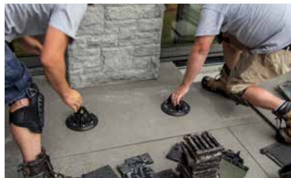
Use a vacuum suction cup lifter for easier and quicker installation
