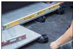
BlackJack® OneStep Extenders provide height extension up to 4.1" (104mm).
