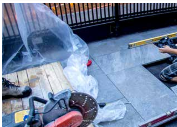
Provide proper protection of pre-existing site conditions during installation (ie. wet cutting residue).
