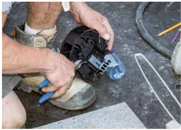
Spacer tabs are easily removed or trimmed when necessary. Spacer tabs should never extend beyond the finished surface.
