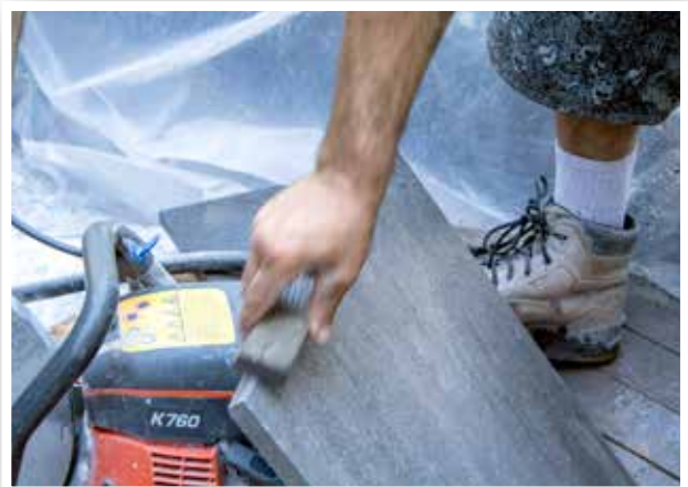
Softening the sharp cut edge with a grinding stone.
