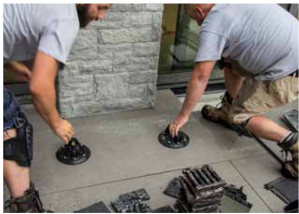
Placement of slab using hand held suction tools.
