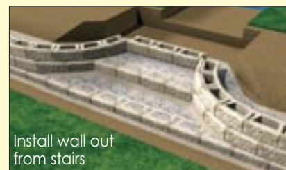
Install next stair riser
