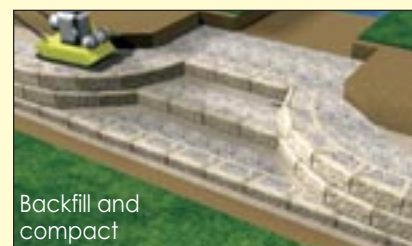
Install wall out from stairs
