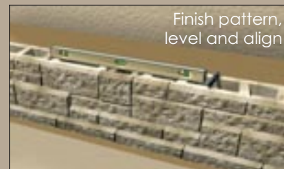
Compact on block and behind
