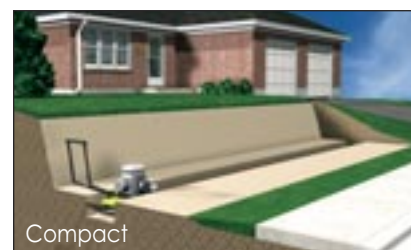
Install drain pipe, wall rock and level
